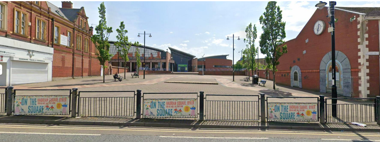
Google Street View Image of Hadrian Square and part of the existing guardrail
